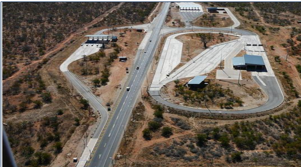
Figure 2.3: Aerial View of the Musina Traffic Control Centre
